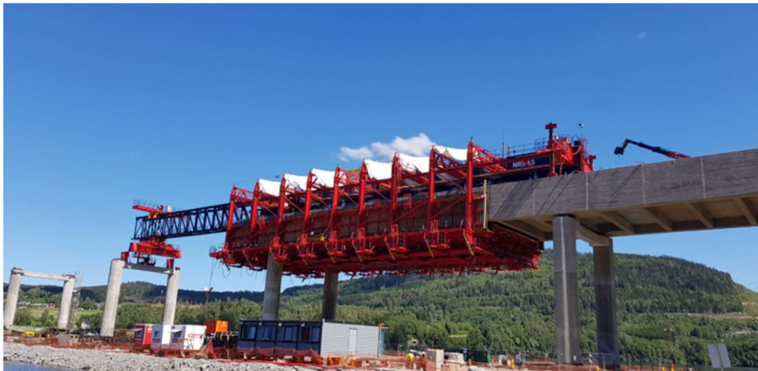
Figur 2-14 Moveable scaffolding system (MSS). Foto: NRS Bridge Construction Equipment
