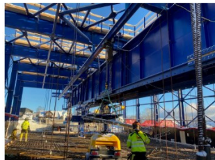
MSS over the railway
