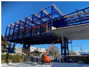
Movable Scaffolding System - MSS
